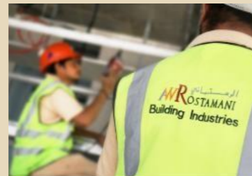
INTERIOR FIT OUT
